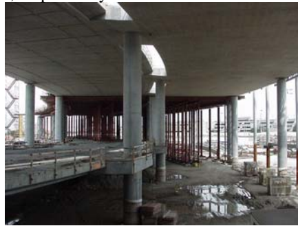
Figure 3 – Partially Completed Section
